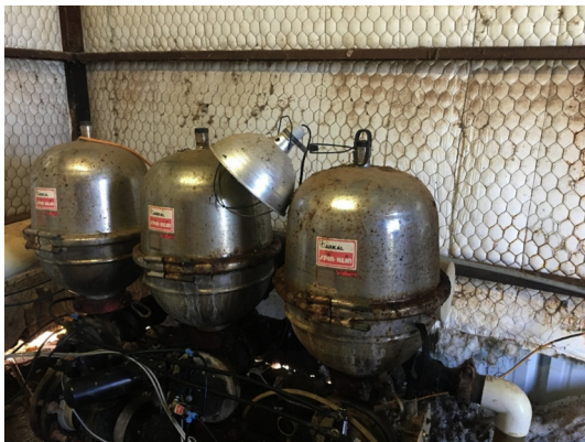
Fig. 2. Disk filtration system for Treated Wastewater: Amiad Arkal Spin Klin Filter with 120 mesh and 130 \mu\text{m} disk size.
