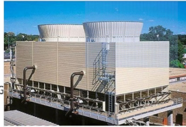
Figure 2 a) Induced draft cooling tower
